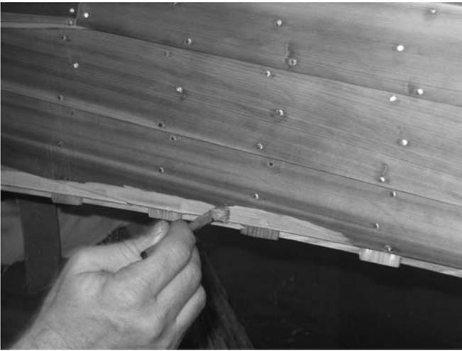
*Figure 1. Applying the adhesive along the top half-inch of the planking. Two coats of adhesive will assure a good bond.*
